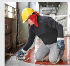
Sl. 8 Nanašanje SikaTransfloor®-352 (SL/ST)
