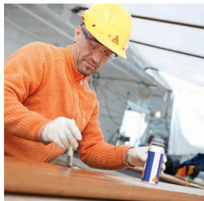
Sl. 10 Skrbno in previdno nanašanje Sika® Primer-290 DC ali Sika®MultiPrimer Marine
