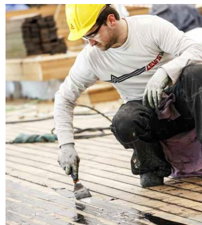
Sl. 19 Glajenje stikov s Sikaflex®-290 DC PRO
